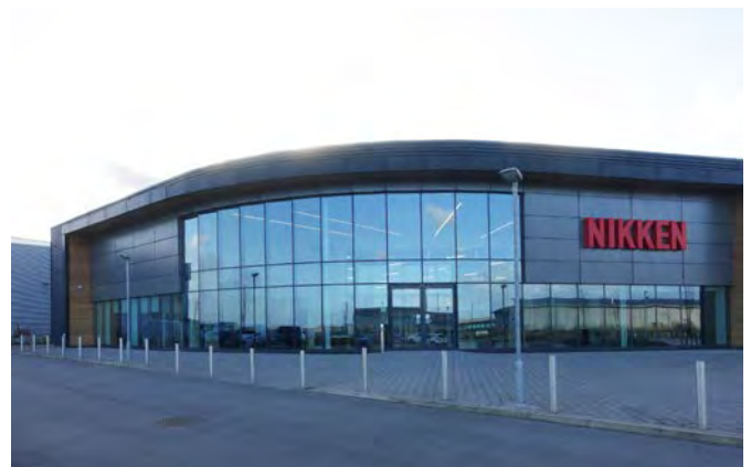
Figure 45. 'Front of house' offices expressed as separate mass to the main works, with curved glazed facade.
