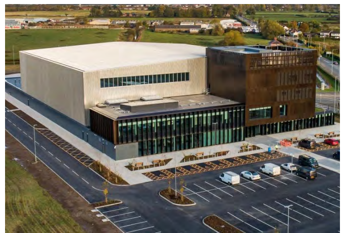
Figure 8. Hard and soft landscaping used to separate vehicular routes and areas of car parking from building frontages.
