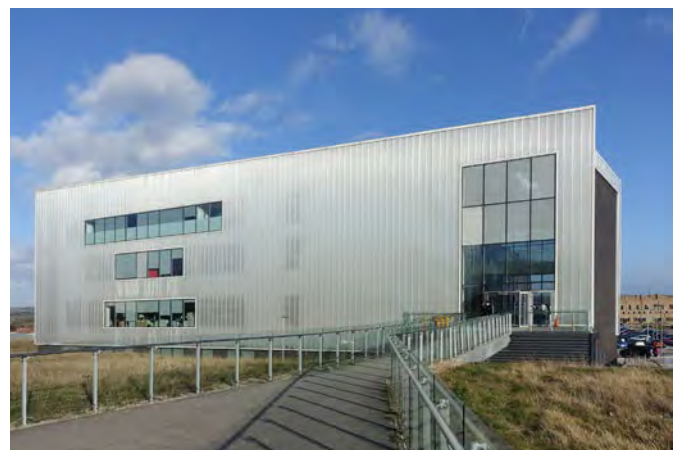
Figure 10. Pedestrian level access bridge to the building frontage separated from lower level service yard and car parking to the rear.
