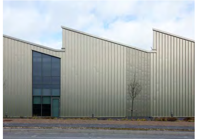
Figure 27. The ‘sawtooth’ profile expresses the function of providing north light within the deep-plan manufacturing space. The south facing sloping sections can be used for roof-mounted photovoltaics.
