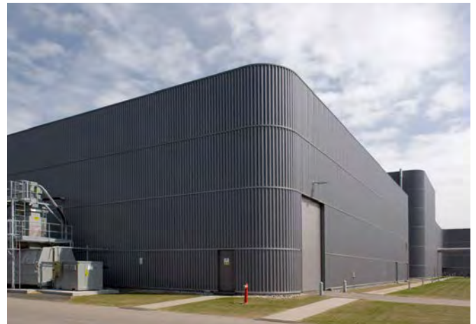
Figure 38. Subtle features (such as curved corners) can soften the impact of a singular cladding material applied to a large industrial volume.
