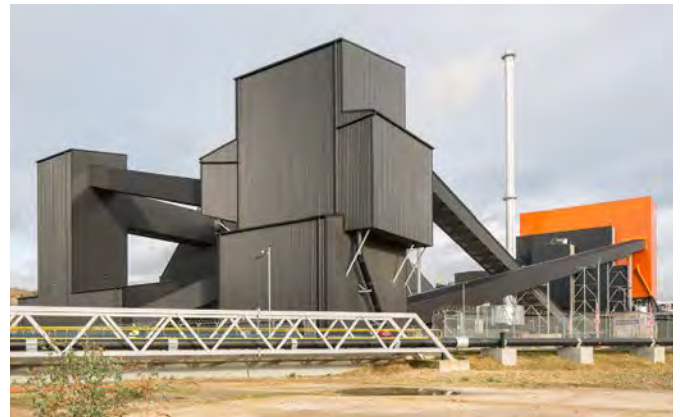
Figure 40. External processing plant can take a variety of forms that express the function of the industrial activity and provide visual interest.
