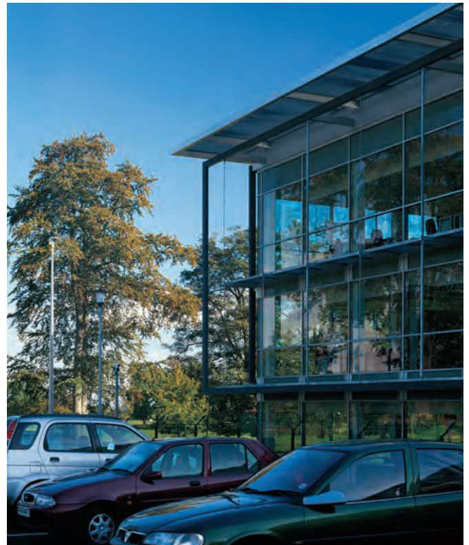
Figure 51. A fully glazed facade of office accommodation with over-sailing roof and brise soleil.
