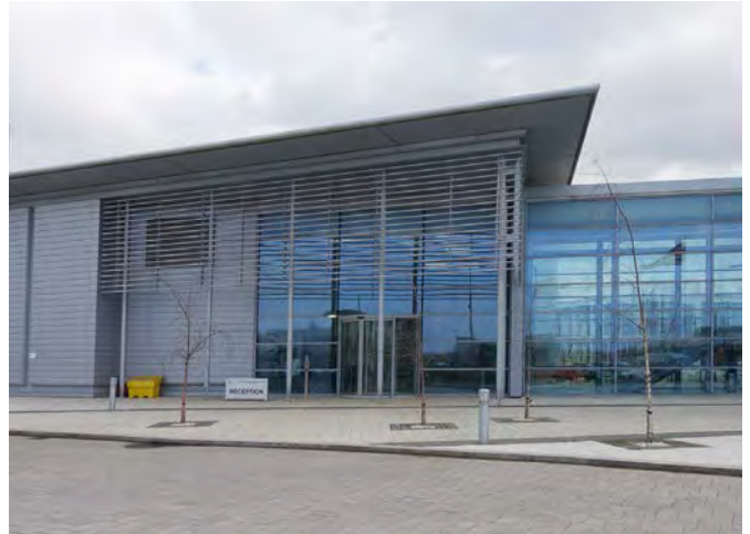
Figure 29. A building entrance expressed through roof profile, over-sailing roof canopy and large area of glazing with brise soleil.
