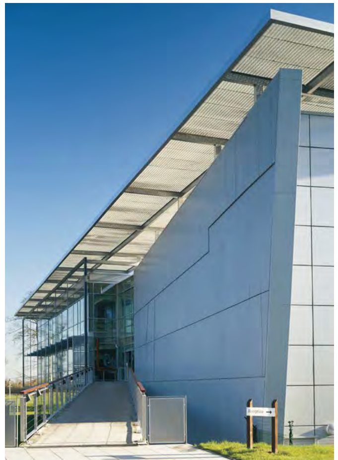
Figure 49. Architectural expression of a building entrance and frontage.
