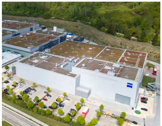
Figure 30. The use of green roofs on industrial buildings can provide a range of benefits including biodiversity contribution and reduced water run-off rates.
