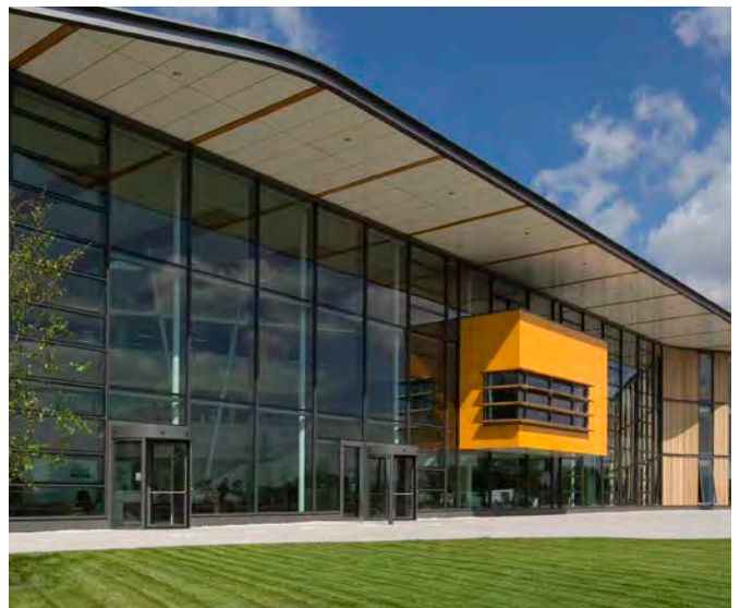
Figure 31. Colour tends to be most effective when used on selected features such as soffits, reveals, or projecting elements.
